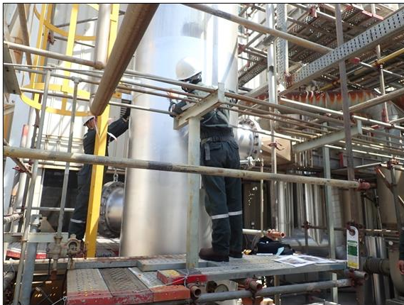
Fitness for service assessment on burning equipment.
