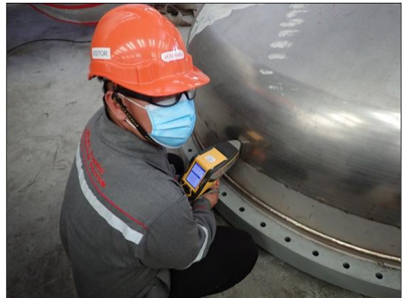
Identify material for newly fabricated equipment using positive material identification.
