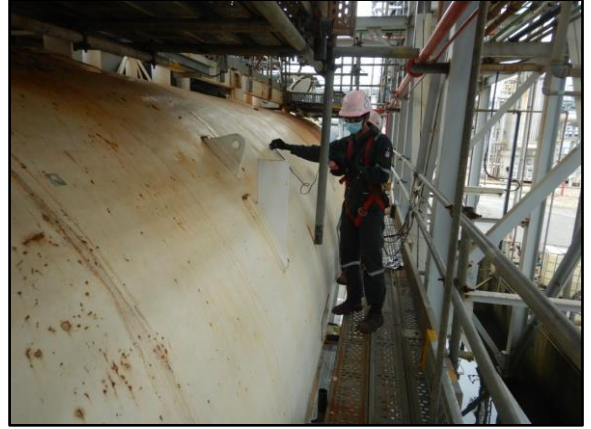
Thickness measurement on pressure vessel using ultrasonic testing.
