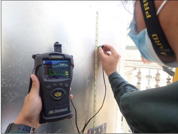
Thickness measurement on grid using ultrasonic testing.
